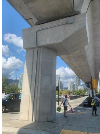
Fig. 1: An example of a C-bent column to allow pedestrian access
